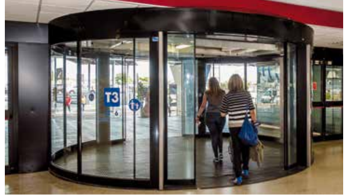
Airport - Ronda composed with two large semicircular Lowered Arch
