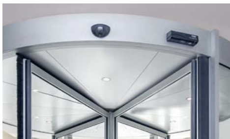
Aluminium sheet inspection ceiling and spotlights
