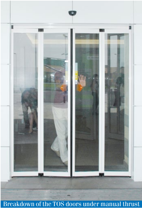
Breakdown of the TOS doors under manual thrust
