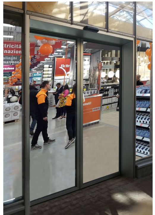
RID on automatic door with thermal break profiles
