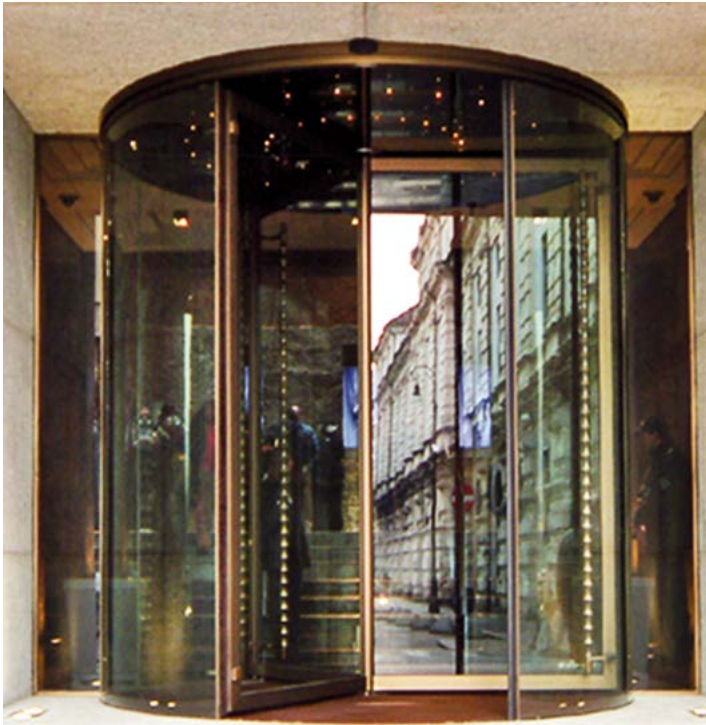
Ponzi Vitrum - Entrance with glazed canopy illuminated with LED
